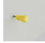
To insert the drywall anchors, use a screwdriver to push and turn the anchor clockwise until flush. Remount track with screw into anchors.
