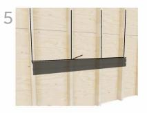
Mark lines vertically to the full height of the 30" display and recheck stud alignment.
