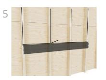
Extend lines vertically to the full height of the 36" display and recheck stud alignment.
